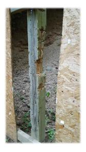
We are also spending significant resources repairing the posts and boards that support the target backer boards on all shooting ranges. We ask all members to make sure targets are mounted at least 4 inches away from the backer supports to avoid hitting upright posts and the 2X4 horizontal supports. They are especially difficult to replace.
