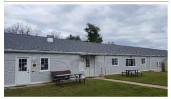
Storms over the past year had blown away shingles and compromised our roof. New shingles were installed that have a 50 year service life.
