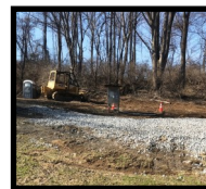
Area Near Completion of Landing
