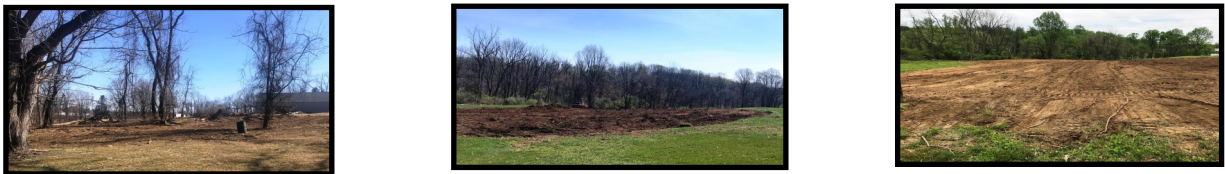
Range at Completion.
