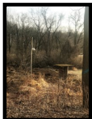
Area at Start of Landing Construction
