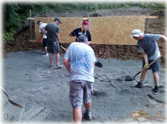
Adjusting the grade on the 15 yard range.
